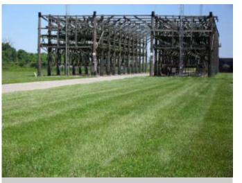
This is the manual antenna switching gear. There were 23 antennas, all switched by hand. Any of the six transmitters could be connected to any of the antennas to meet the needs of direction and frequency. The antennas covered one square mile. Both rhombics and curtain arrays were used.
