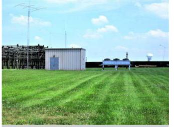
The dummy load building. That's right, a dummy load so big it needed it's own building. Those three air conditioning units were necessary to keep it cool.
