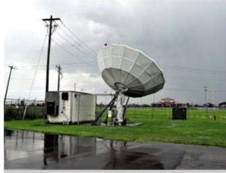
One of two satellite dishes, installed early 80's. Prior to that, VOA programming was piped in via AT&T " long lines Using Six primary lines, one for each transmitter, and six backups incase of a line failure.
